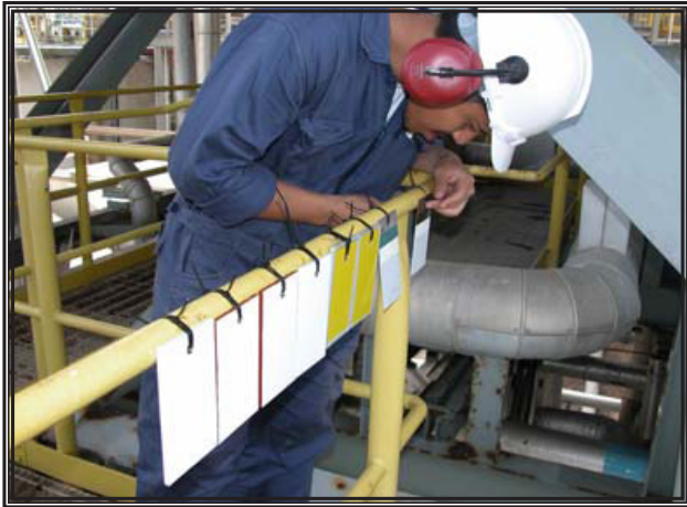
Installation of test coupons at site for evaluating best coating materials.
