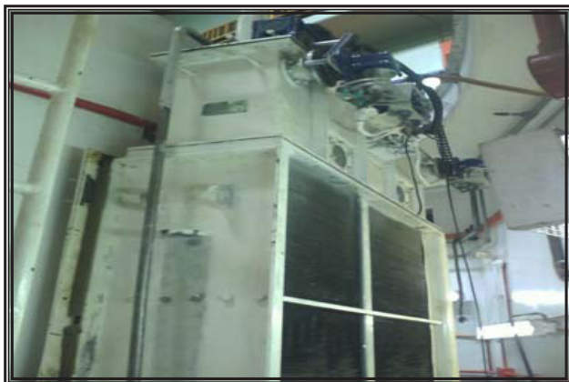
View of the cleaning brushes at rest position (just above the tubes)
