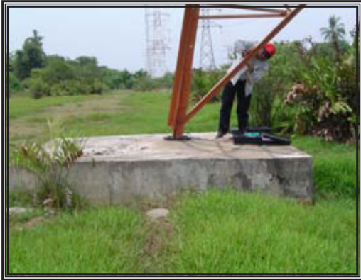
Ishak Che' Pee inspecting the tower and making TFR measurement preparations
