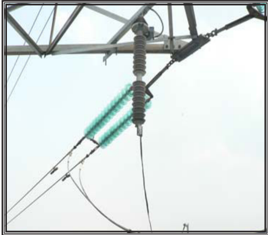
ABB TLA (PEXLIM) installed on Balakong to Serdang 132kV line
