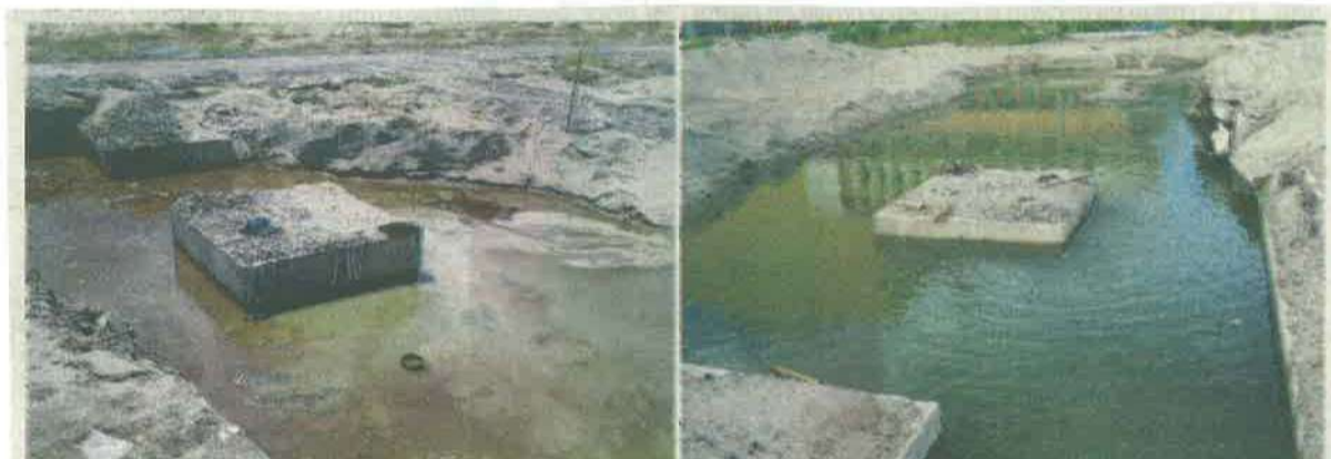
Before (left): Water contaminated by transformer oil spillage at the Perai Power Station in Penang. After: Clean water after the bioremediation process.
